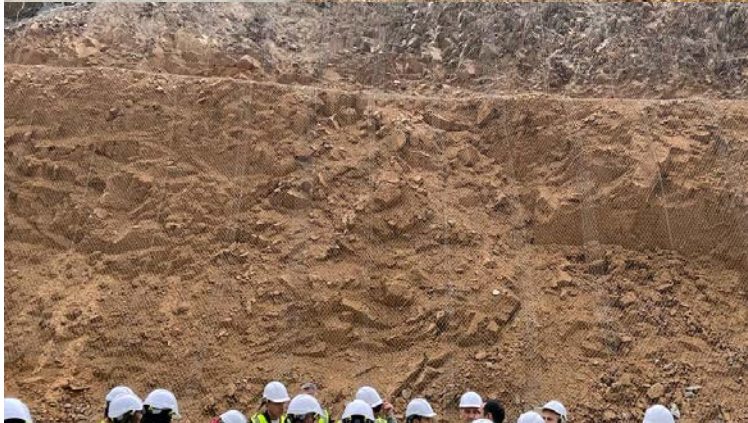
Wire mesh screen attached to cut face to stop small rocks from causing danger to people and machinery.
