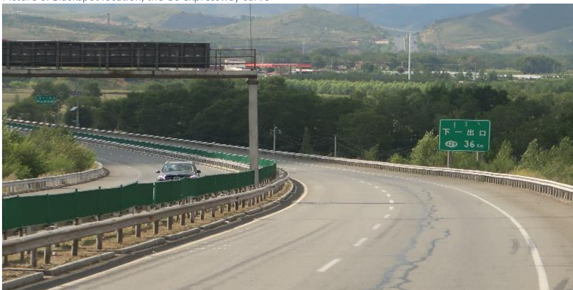
Picture 6: Blackspot location, the G6 expressway curve
