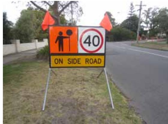
Messages can be changed quickly to accurately reflect the type of works underway at the time. Regulatory signs must conform to national road rules so they can be enforced.
