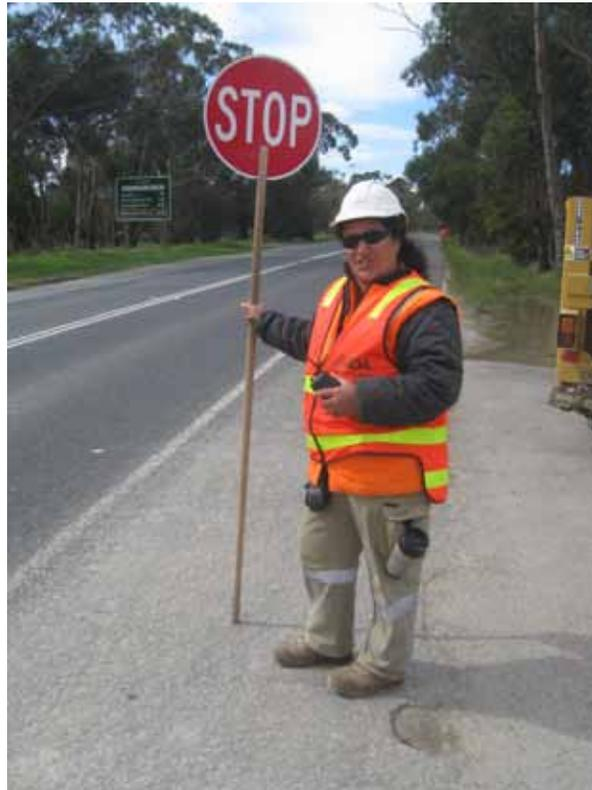
Workers and traffic controllers must be provided with personal protective equipment suited to the climatic conditions. It should include a high-visibility jacket or vest, which offers high-visibility for daytime and good reflectivity for nighttime conditions.
