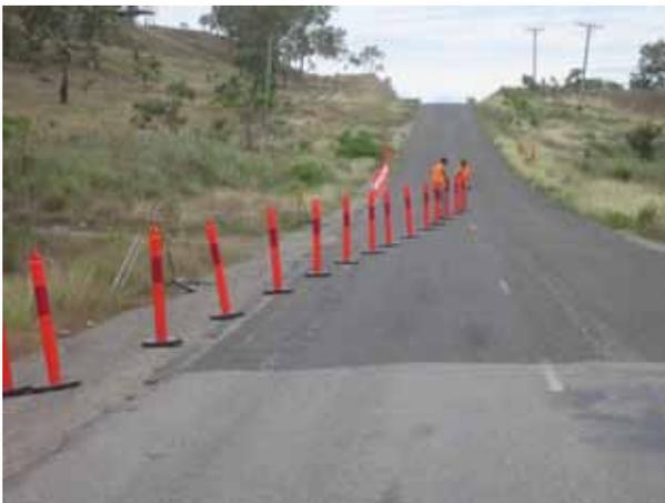
Traffic cones and bollards are best placed 5 meters apart in a taper.
