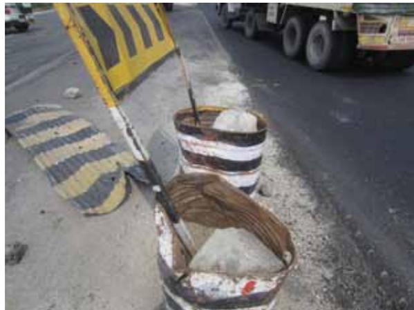
Good delineation is essential at road worksites, but it must be forgiving and reflective. Concrete blocks inside painted barrels are hazards.
