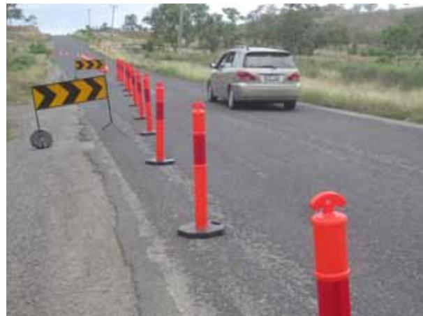
Devices used to delineate traffic paths are to be highly visible, reflective, and forgiving if struck. Plastic bollards, 1,200 millimeters high are an excellent form of delineator. They have a heavy base to keep the bollard vertical under most weather conditions.
