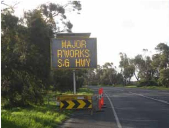
An example of a trailer-mounted variable message sign located just off the shoulder of a rural highway with a speed limit of 100 kilometers per hour (driving on the left side).
