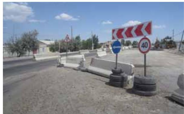
These regulatory signs are too close to the work zone. The concrete barriers are not secured together, and are roadside hazards.
