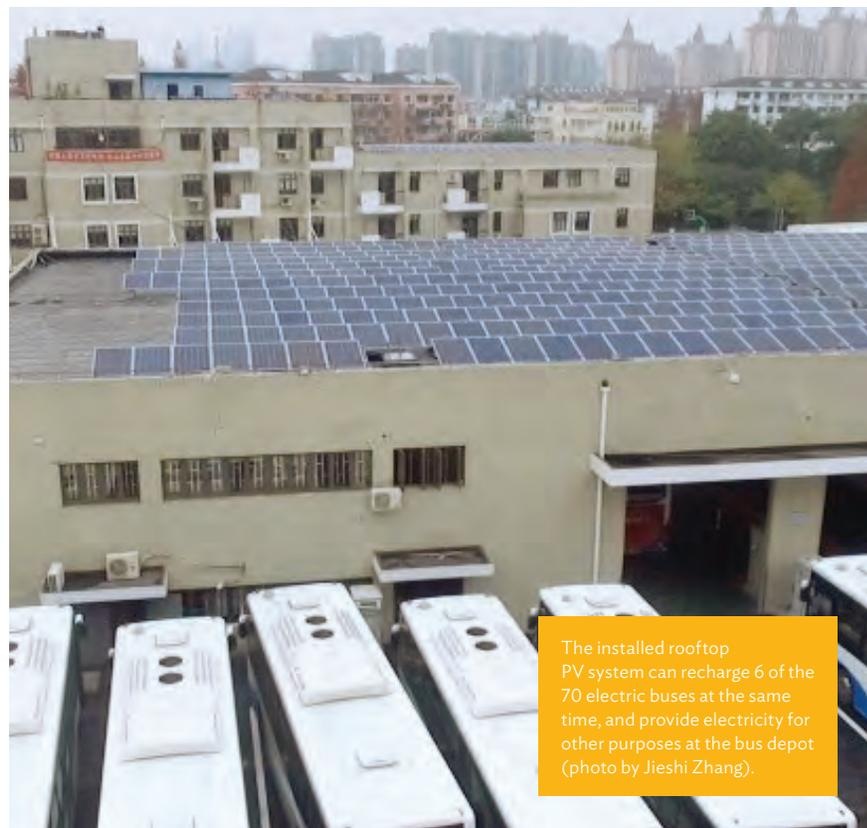
The installed rooftop PV system can recharge 6 of the 70 electric buses at the same time, and provide electricity for other purposes at the bus depot (photo by Jieshi Zhang).
