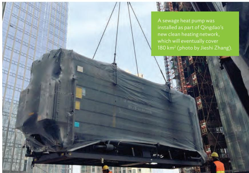
A sewage heat pump was installed as part of Qingdao's new clean heating network, which will eventually cover 180 km<sup>2</sup> (photo by Jieshi Zhang).
