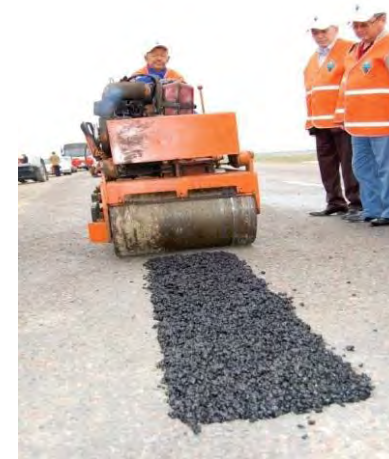
Patching with application of MAC-asphalt
