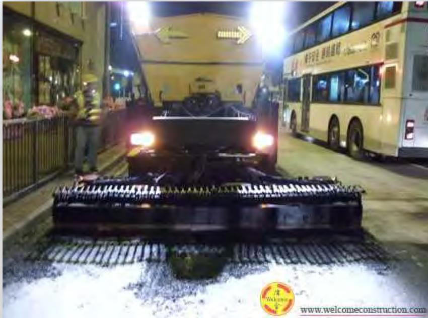
Step 3 - Some existing surface were removed due to its serious oxidation and contamination by road marking
