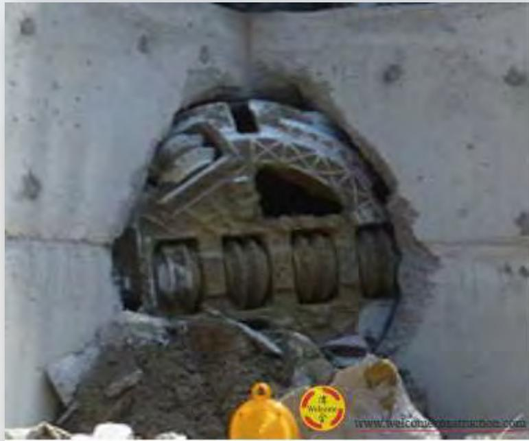
Pipe jacking unit by hydraulic jack
