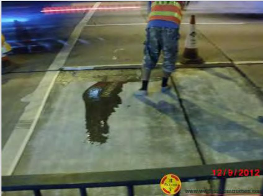
Mix the Matacryl resin and apply to the surface (Step 4)
