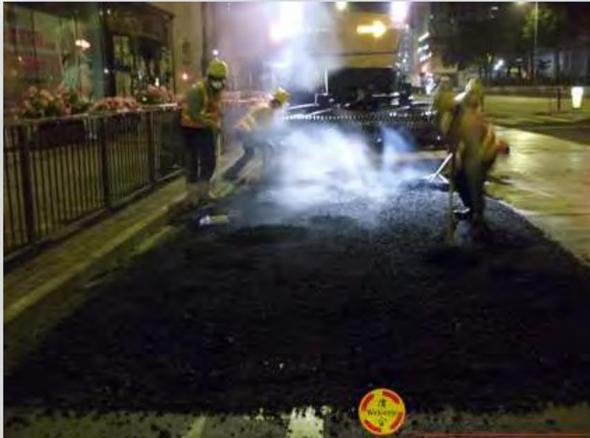
Step 5 - Proper grading and compaction to achieve a new surface before road opening
