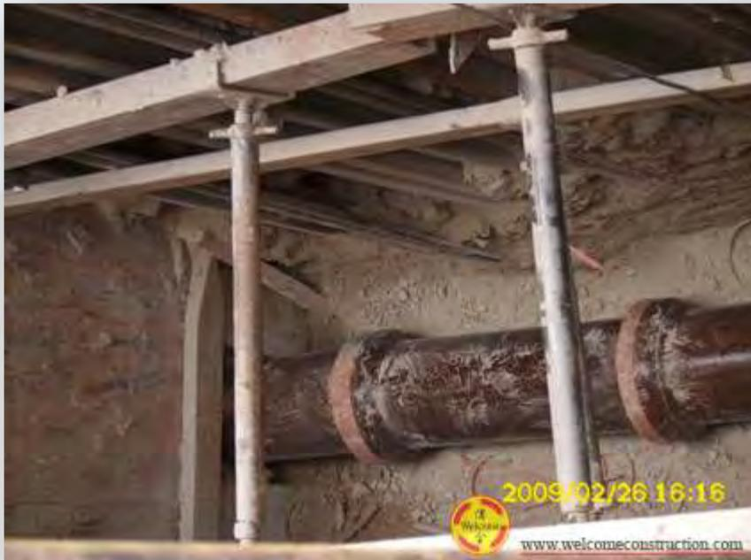
Pipe ready for concrete surround and backfill
