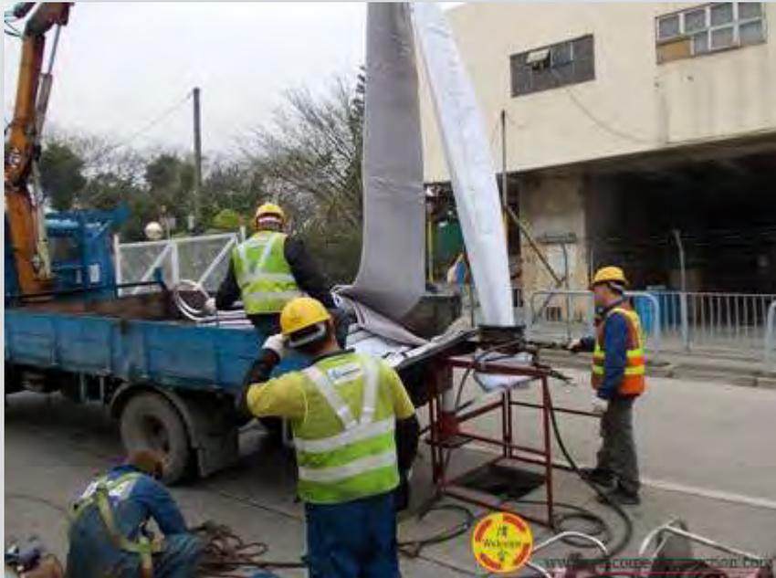
Liner to be blown up to keep intact to the inner side of the cracked concrete pipe and cured by steam
